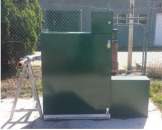
Standpipe with pipe and instructions panel
