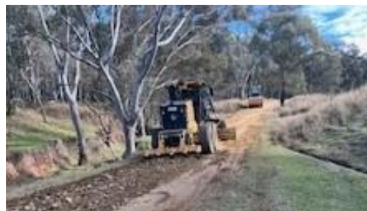
Above: Resheeting work on Yabtree Road in Gundagai
