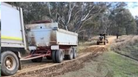
Above: Resheeting work on Yabtree Road in Gundagai
