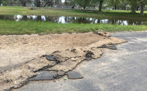
Landon Street Gundagai. Flood waters from Morley's Creek have damaged the road surface. Highlighting the dangers of driving through flood waters. This damage was revealed after the water receded. If it's flooded, forget it!!
