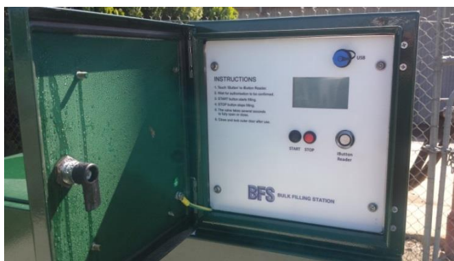
Standpipe with pipe and instructions panel
