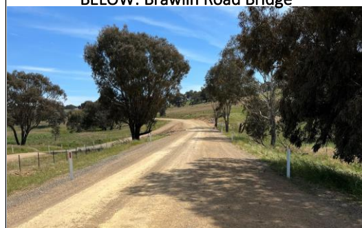
BELOW: Brawlin Road Bridge
