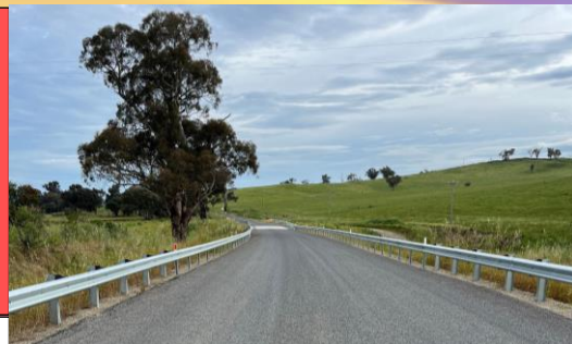
ABOVE: The new Burra Road Bridge.
