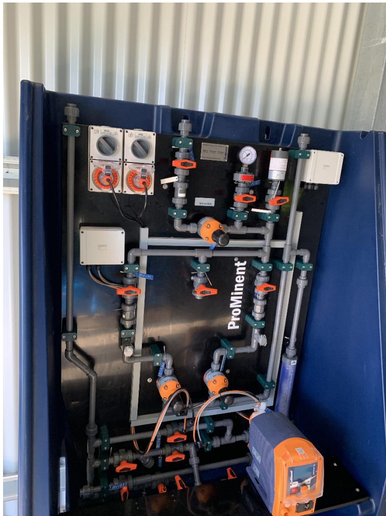
Figure 3 - Chlorinator
