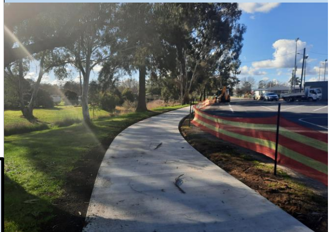
Above: CGRC crews are constructing footpath/cycle path along Muttuma Creek adjacent to the car park of Ex Services Club in Cootamundra. After construction is completed, this shared footpath/cycleway along the creek will link Parker and Wallendoon Streets and will provide a safer off road travel route for pedestrians, gophers and cyclists.
