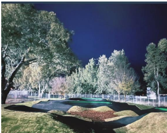
Cootamundra's Pump Track nears completion and will be Opening Soon!
