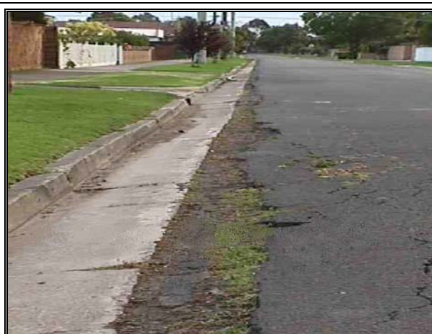
Condition 6 Movement and concrete breakdown
