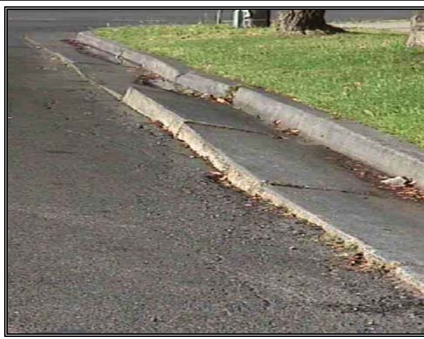
Condition 9 Extreme movement and lack of function
