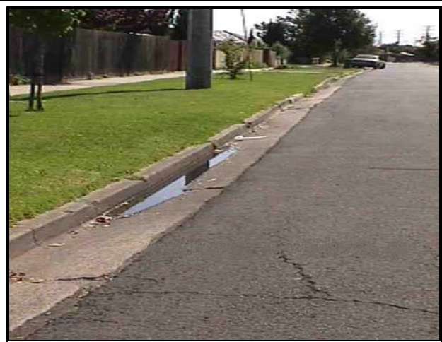
Condition 8 Large movement and holding of water
