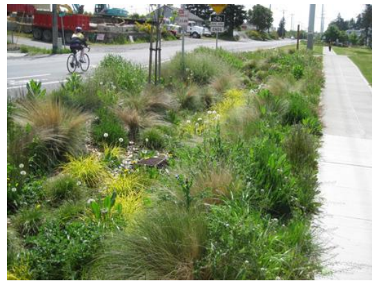
Figure 18: Raingardens are spaces which allow for water of between 200mm to 500mm to settle for a short period after intensive rainfall before draining into the stormwater network. Generally a mesh or filter material is used to ensure that soil remains and does not enter the stormwater network: source Melbourne Water.
