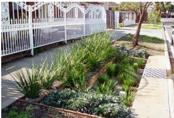
Figure 18: Raingardens are spaces which allow for water of between 200mm to 500mm to settle for a short period after intensive rainfall before draining into the stormwater network. Generally a mesh or filter material is used to ensure that soil remains and does not enter the stormwater network: source Melbourne Water.
