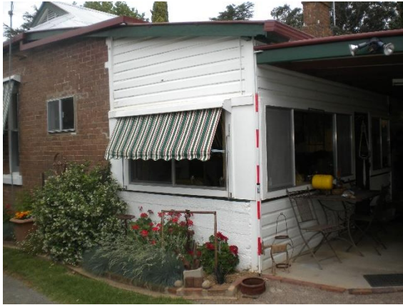
Plate 29. White weatherboard extension at the rear of the house.
