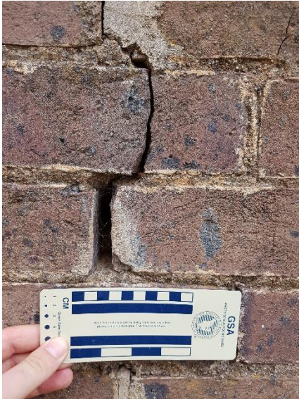
Plate 90. Detailed view of cracking within the mortar of the Church walls.
