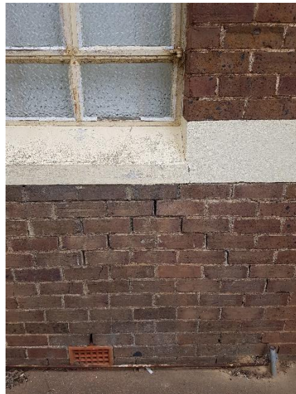
Plate 89. Cracking along the mortar in the wall and some deterioration of paint along windows.
