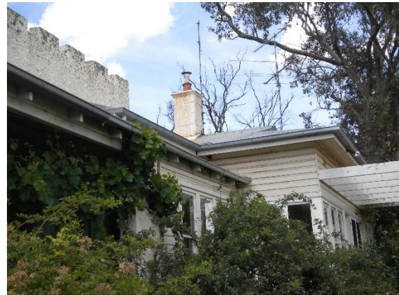
Plate 235. Original battlement roof contrasting with the pitched roof of the weatherboard extension.
