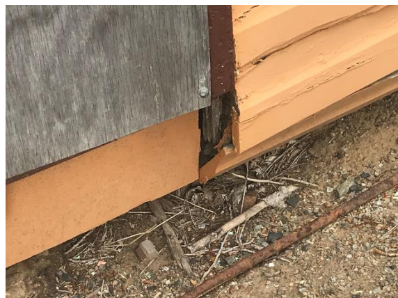
Plate 203. Damage and rot to the wood join.
