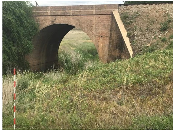
Plate 207. Brick arch Underbridge with steep incline up to railway track.
