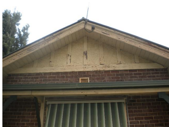
Plate 45. Gable roof at the front of the house. Noticeable paint loss and degradation on the guttering and decoration.
