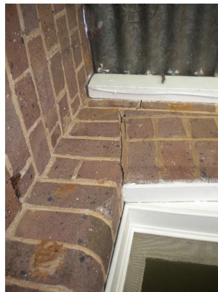
Plate 38. Some minimal cracking of the mortar from the window to the roof
