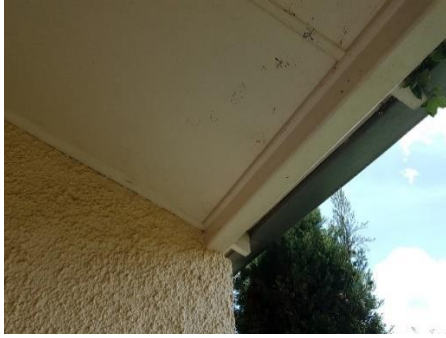
Plate 220. Verandah ceiling with mould growth and inhabited by invertebrates.
