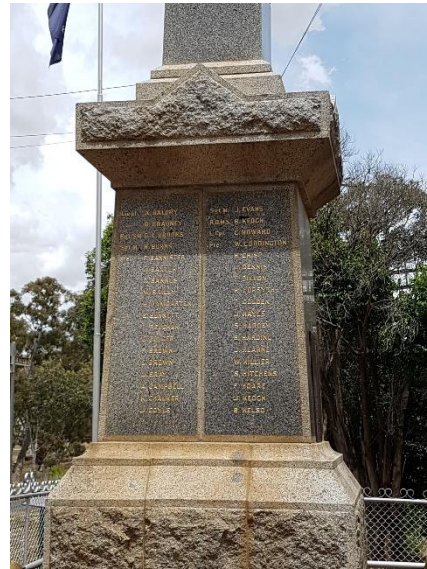
Plate 79. Obelisk constructed of grey harcourt granite.
