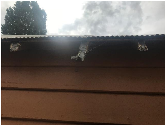
Plate 200. Damage to roof and guttering
