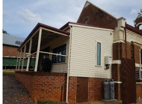
Plate 149. Weatherboard extension to the rear of the Church.
