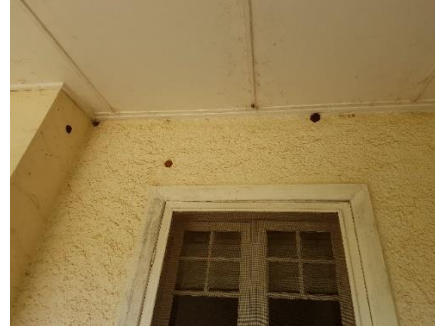
Plate 221. Wasp casings present of ceiling and walls of verandah.
