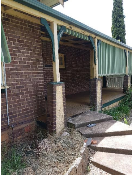
Plate 47. Front entrance to the home. Paint degradation on the guttering.
