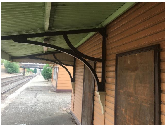
Plate 192. Metal brackets supporting roof.
