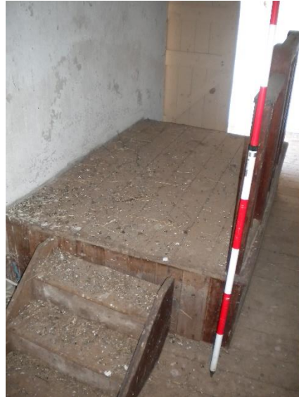
Plate 179. Dust, mould and bird droppings.
