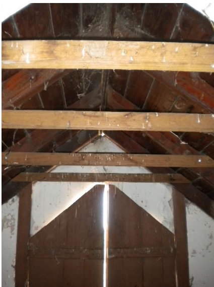
Plate 172. Significant paint deterioration. Numerous cobwebs present as well as bird droppings.
