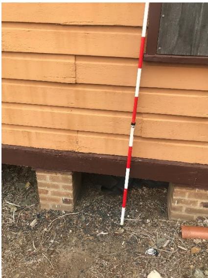
Plate 196. Weatherboard structure on brick stilts.
