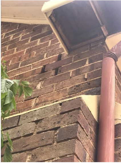
Plate 102. Separation of bricks and loss of mortar towards the guttering
