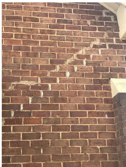
Plate 106. Crack remediation from the wall up to the roof in a diagonal direction.
