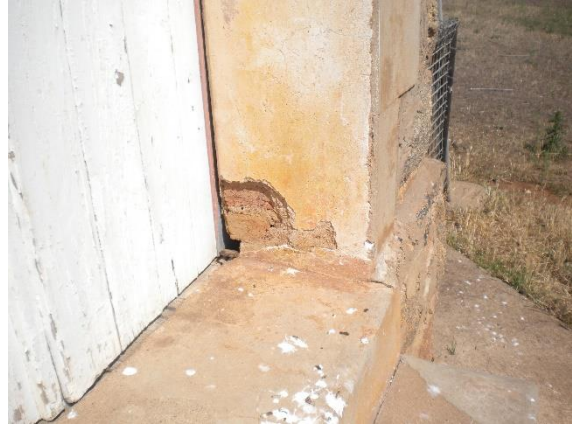
Plate 167. Damage to the stone surrounding the entrance door and deterioration of paint.
