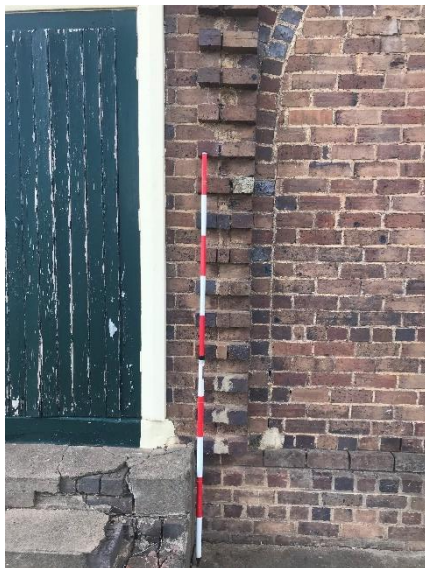
Plate 100. Brick detailing on the northern façade of the Church and damage to rendered bricks used to enter and exit the back door of the church.
