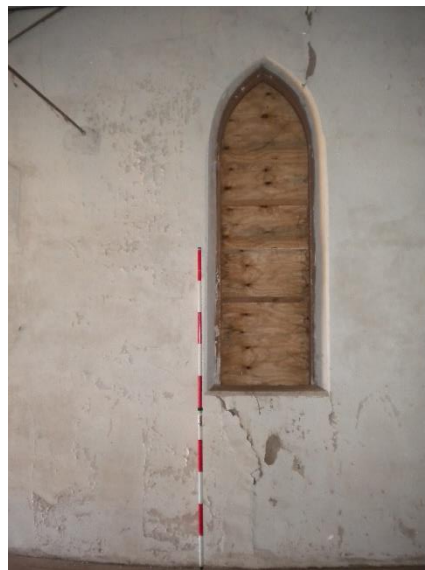
Plate 173. Peeling paint and bordered up window.
