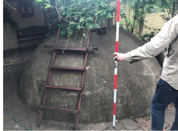
Plate 245. Well covered with a concrete dome.
