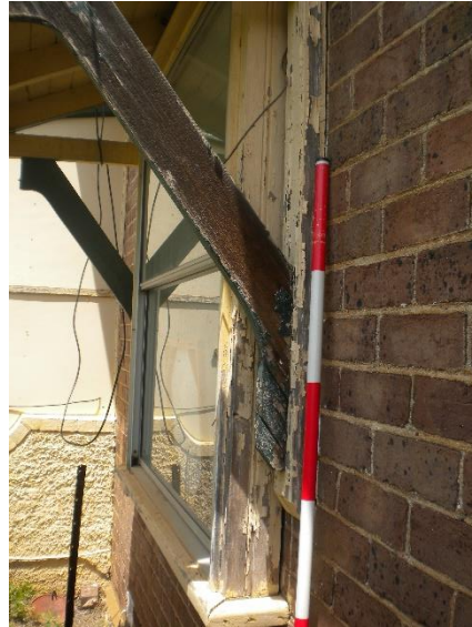
Plate 60. Wooden awning over window at the front of the house. Significant loss of paint.
