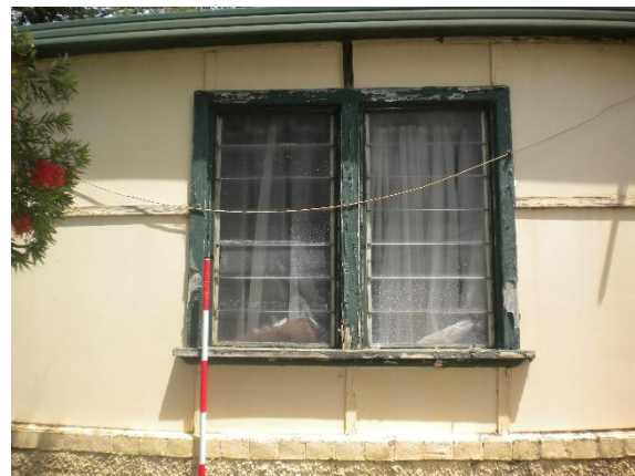
Plate 62. Significant paint degradation on window frame.
