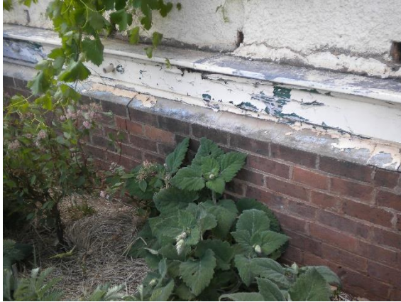
Plate 232. Significant deterioration and cracking of paint at the front of the house.
