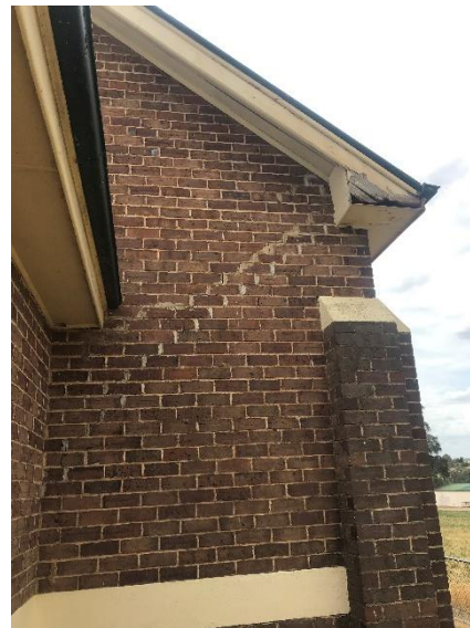
Plate 105. Crack remediation from the wall up to the roof in a diagonal direction.
