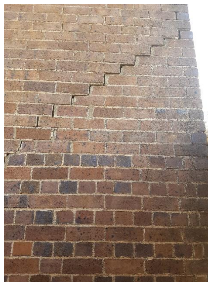
Plate 130. Some movement of bricks and cracking of mortar in a diagonal direction.
