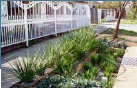
Figure 18: Raingardens are spaces which allow for water of between 200mm to 500mm to settle for a short period after intensive rainfall before draining into the stormwater network. Generally a mesh or filter material is used to ensure that soil remains and does not enter the stormwater network: source Melbourne Water.
