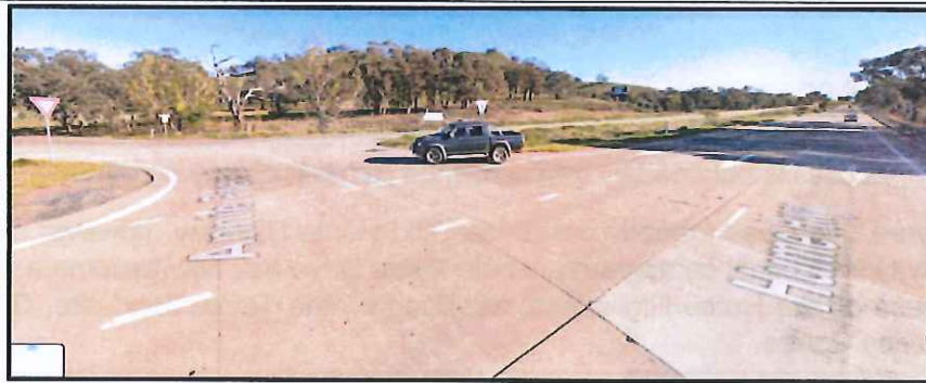
Figure 3.2.3. Image source – Google maps (Street view). Image showing a vehicle turning right at the northern entry point to the Five Mile Precinct. Turning bays allowing for deceleration and stopping before crossing the northbound lanes.
