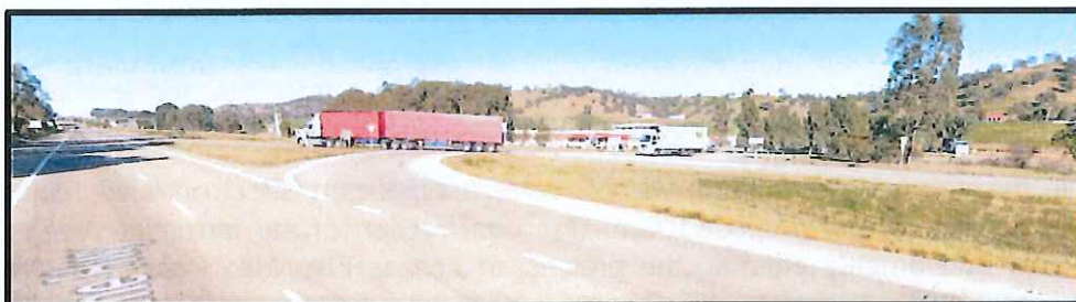
Figure 3.2.2. Image source – Google maps (Street View). Image showing a B-double departing (turning right) from the Shell Service Centre at the southern end to the Five Mile Precinct. Turning bays allowing and merging lanes facilitate safer access for vehicles to re-entering the highway
