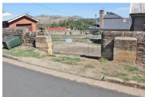
Photo 4: External Boundary wall – north entry
