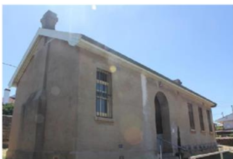
Photo 9: Hospital / Infirmary Block – south façade
