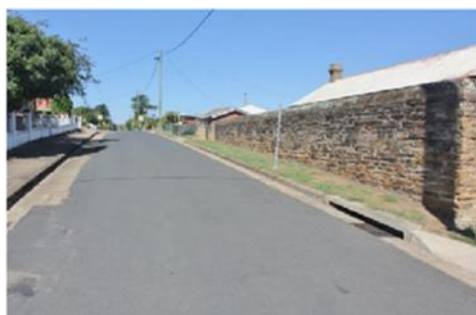
Photo 3: External Boundary wall – north
