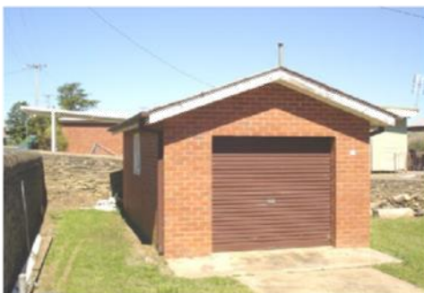
Photo 19: Kitchen Block – east facade
