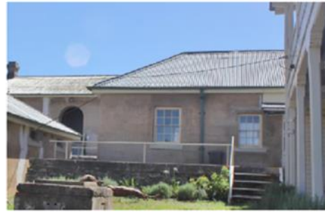
Photo 14: Kitchen Block – south facade
