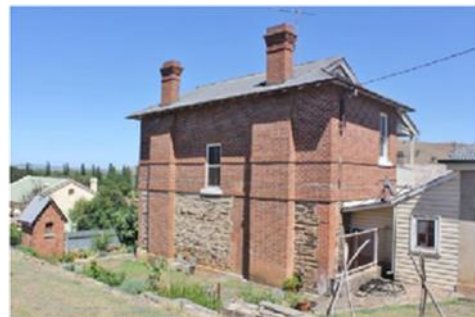
Photo 26: Goalers Residence – east facade
