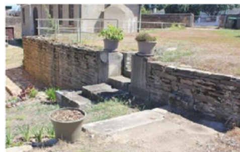
Photo 42: Wall bases, tower plinth & steps
