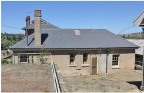
Photo 13: Kitchen Block – north facade
