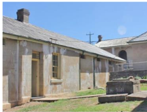
Photo 32: Gaol – east facade & entry
