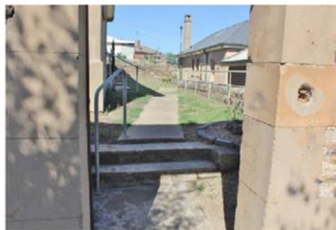
Photo 8: External Boundary wall – main entry
