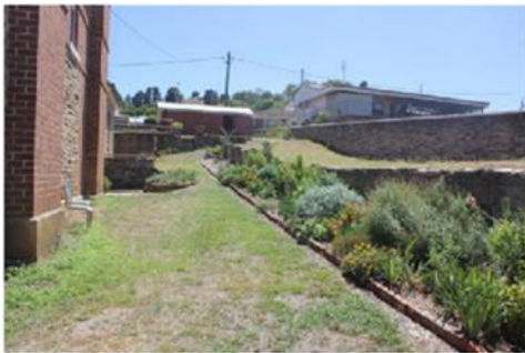
Photo 23: Kitchen Block – east façade
