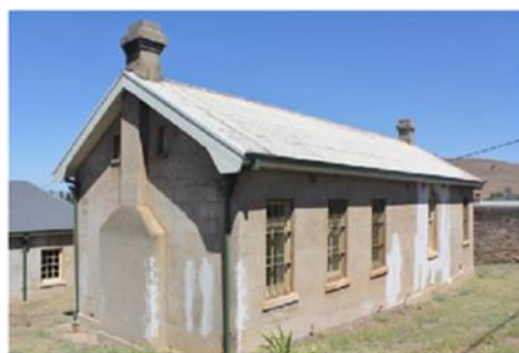
Photo 10: Hospital / Infirmary Block – north facade
