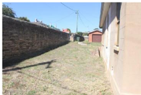
Photo 6: External Boundary wall – north
