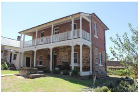
Photo 25: Goalers Residence – west façade
