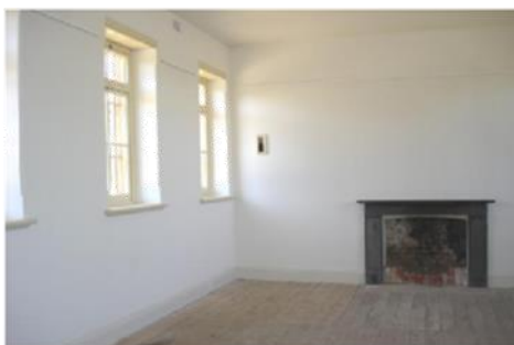
Photo 11: Hospital / Infirmary Block – main room
