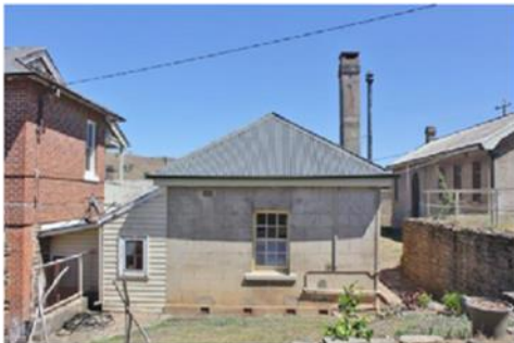
Photo 15: Kitchen Block – east facade
