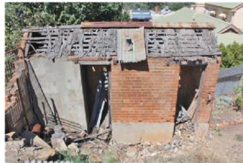
Photo 24: Kitchen Block – east facade
