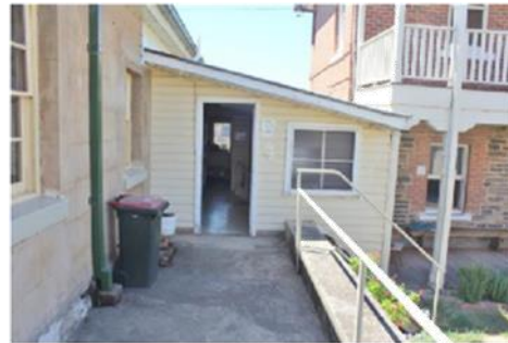
Photo 16: Kitchen Block – west link facade
