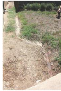
Photo 43: Site drainage – north & court spoon drains
