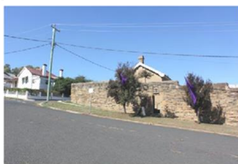
Photo 2: External Boundary wall – north-west
