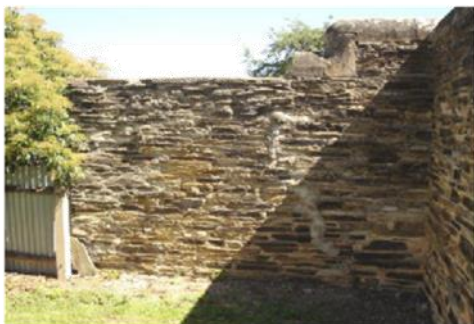
Photo 7: External Boundary wall – south
