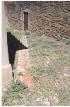
Photo 43: Site drainage – north & court spoon drains
