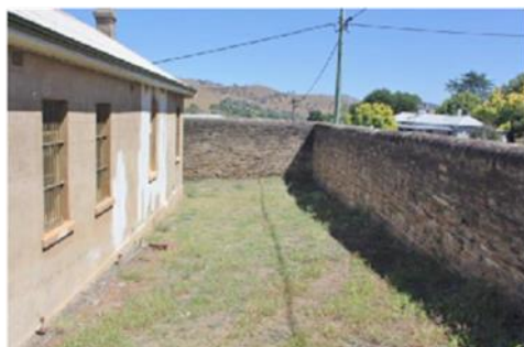
Photo 5: External Boundary wall – north
