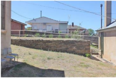
Photo 21: Kitchen Block – east façade
