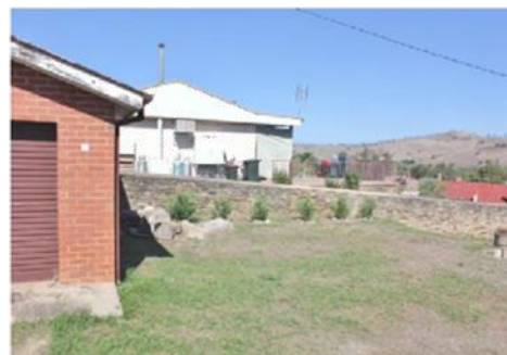
Photo 20: Kitchen Block – east facade
