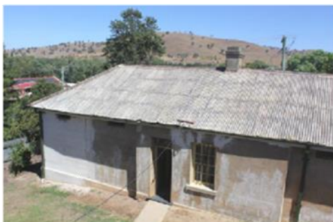
Photo 33: Gaol – east facade & entry
