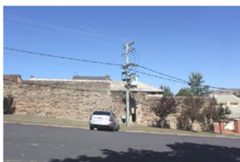
Photo 1: External Boundary wall – south-west
