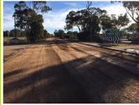
Work is nearing completion on the Burley Griffin Way upgrade through Stockinbingal. The last section of pavement is currently being trimmed with the expectation it will be sealed in the next week. The parking area into the rest area and old Railway Station will be sealed at the same time. The replacement of guard
