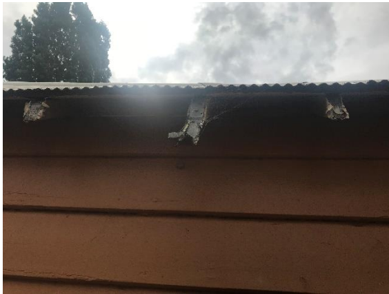
Plate 200. Damage to roof and guttering
