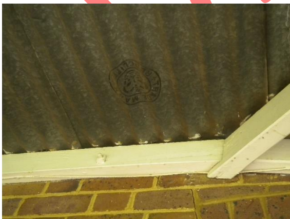
Plate 39. Galvanised roof with Trade mark symbol
