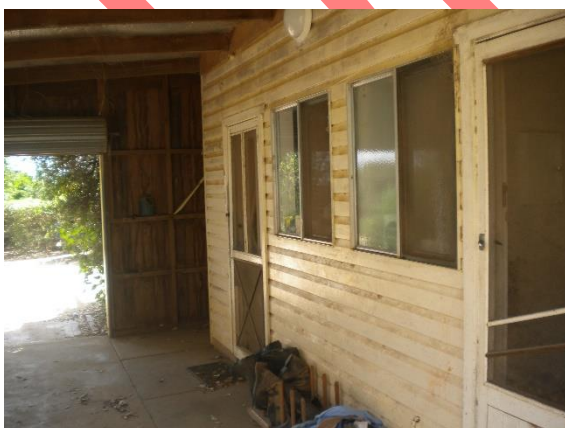
Plate 236. Some deterioration of paint on the weatherboard.
