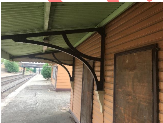
Plate 192. Metal brackets supporting roof.
