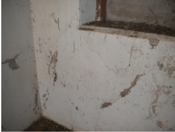
Plate 174. Significant paint deterioration and peel.
