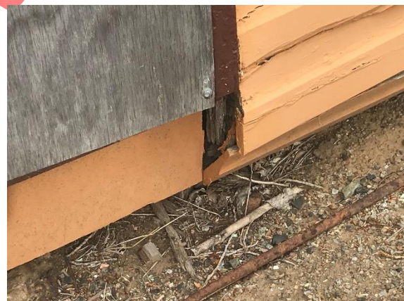
Plate 203. Damage and rot to the wood join.
