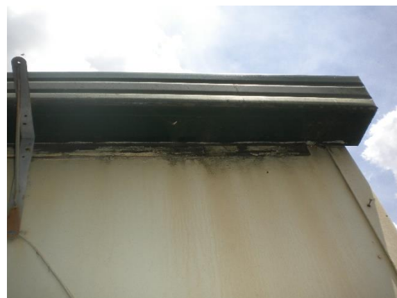
Plate 64. Mould and Mildew growth underneath the eaves of the building.
