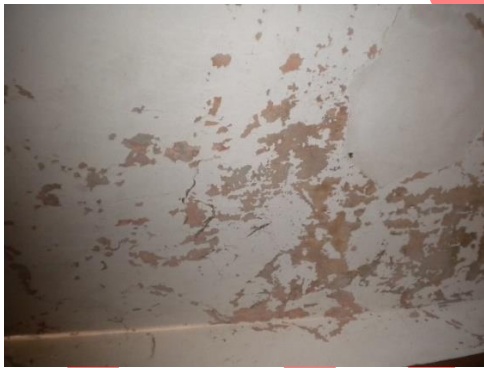
Plate 180. Paint peel and deterioration.
