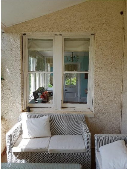
Plate 216. Some minor cracking on the stucco on verandah.
