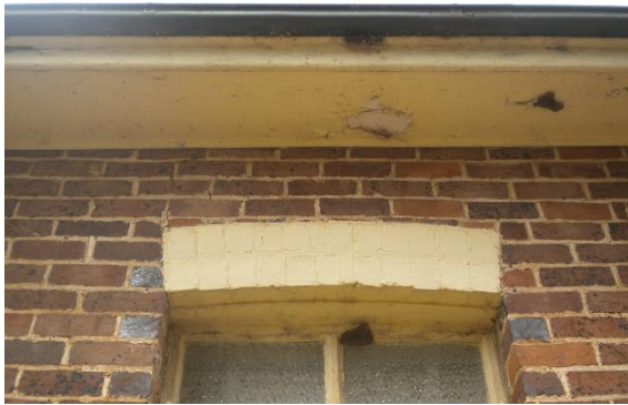
Plate 98. Deteriorated and peeling paint on the eaves and guttering above one of the Church windows.
