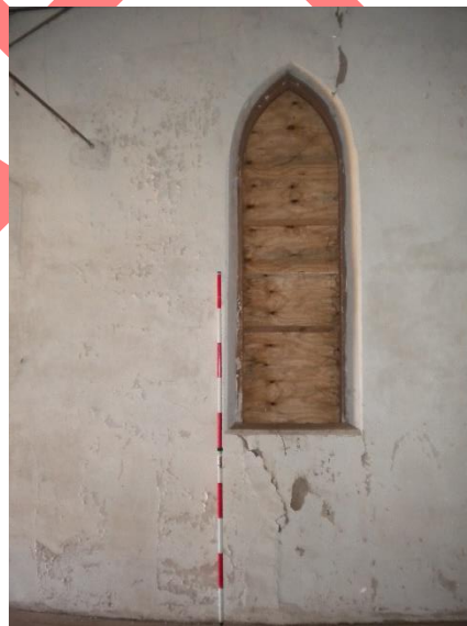
Plate 173. Peeling paint and bordered up window.
