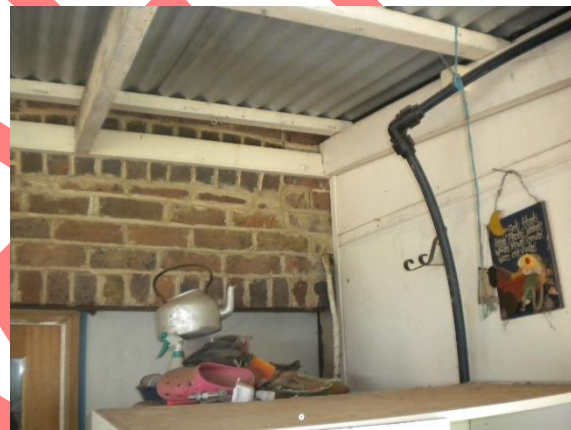
Plate 54. Internal view of the extension. Note the placement of decorative bricks which highlights that a door (or potentially window) was once in place.
