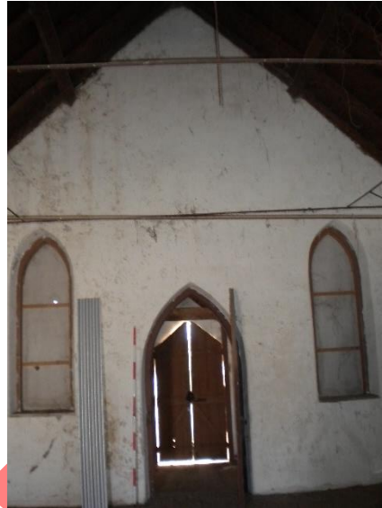
Plate 171. Internal view of structure. Considerable paint deterioration and mould and mildew growth.
