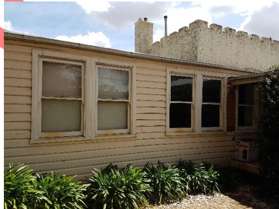
Plate 225. Weatherboard extension to the rear of the house. Some deterioration of paint around windows and on the weatherboard.
