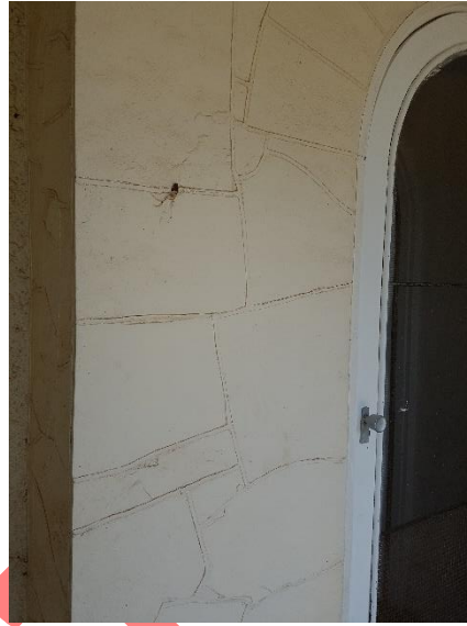
Plate 217. Some mould growth and invertebrate nests present on the verandah.
