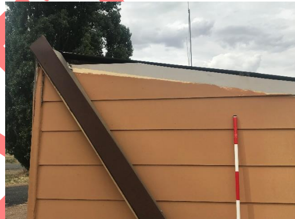
Plate 201. Damage to roof with the guttering pulling away from some areas.
