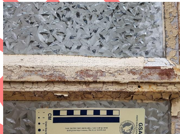
Plate 93. Significant paint deterioration across the window muntin. Paint is flaking off in large sections.
