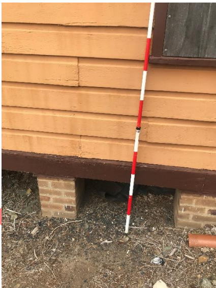
Plate 196. Weatherboard structure on brick stilts.
