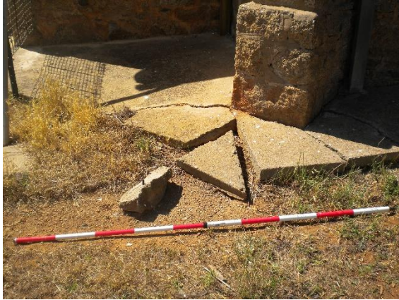
Plate 166. Some cracking and damage to the paving stones surrounding the building entrance.
