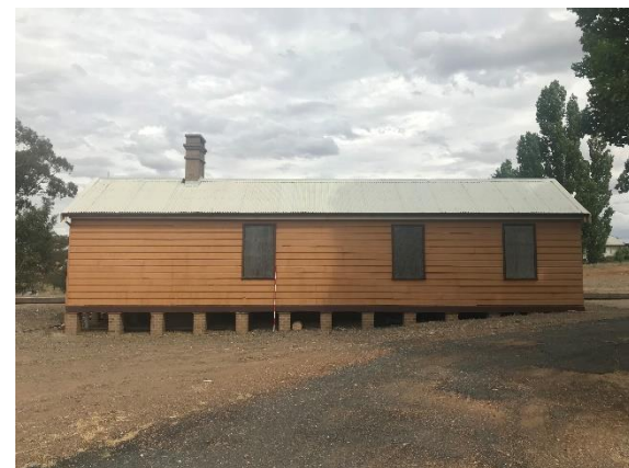
Plate 193. Western façade of the railway building. Brick stilts to compensate for the uneven ground.
