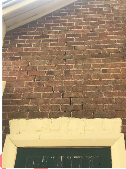
Plate 103. Separation of bricks and loss of mortar above door frame.
