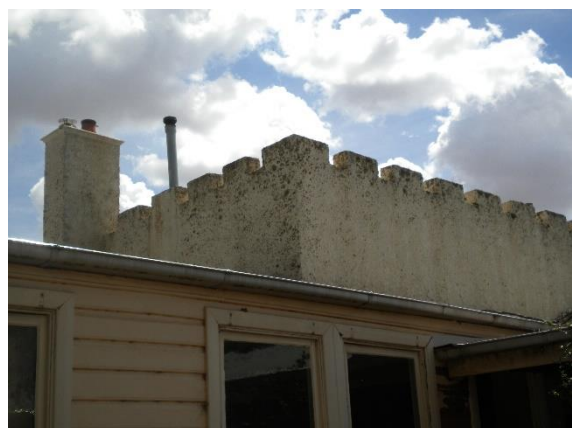
Plate 237. Mould and mildew growth on the upper sections of the battlements.
