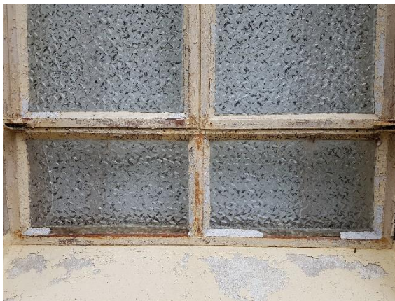
Plate 92. Significant paint deterioration across the window muntin and moulding/trim.
