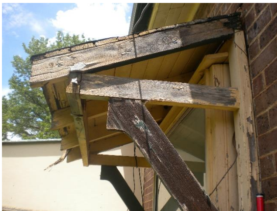
Plate 61. Wooden awning over window at the front of the house. Significant loss of paint.
