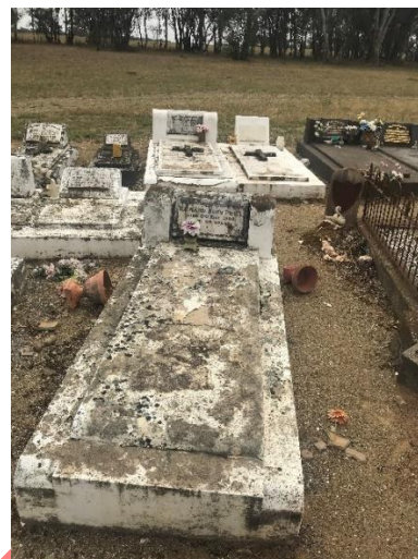
Plate 22. Mould and mildew build up on numerous grave stones.
