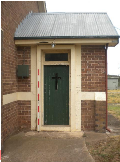
Plate 96. Entrance porch on the southern (main entrance) side of the Church. The section is smaller than the main building and contains a pitched roof of the same slope as the main building.
