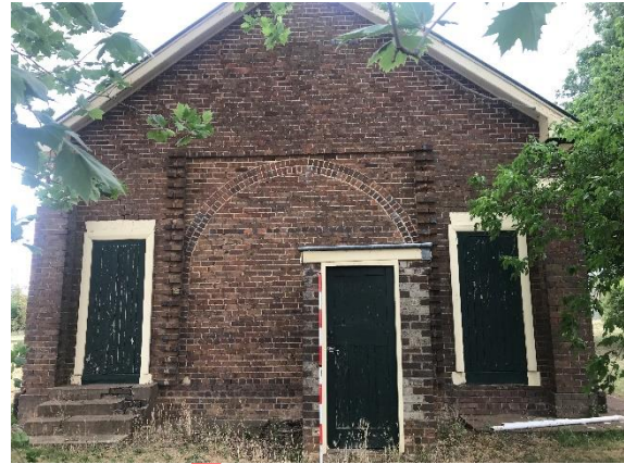
Plate 99. Northern (back) façade of the church. Significant paint deterioration on all three doors.
