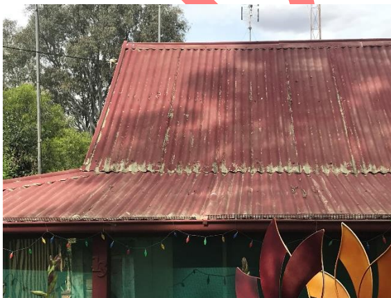
Plate 242. Faded galvanised roof with steep pitch.
