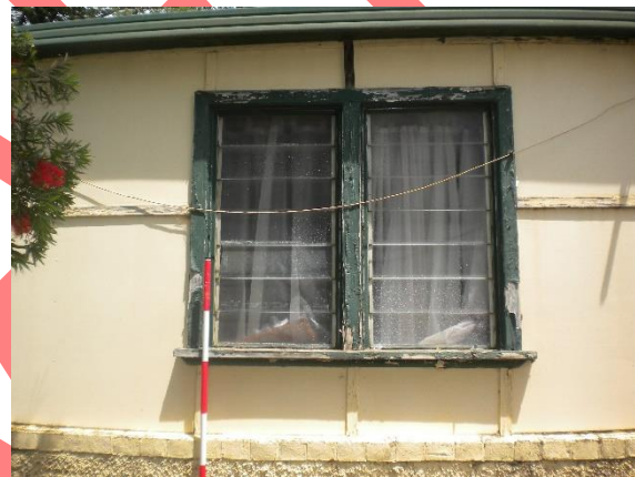
Plate 62. Significant paint degradation on window frame.
