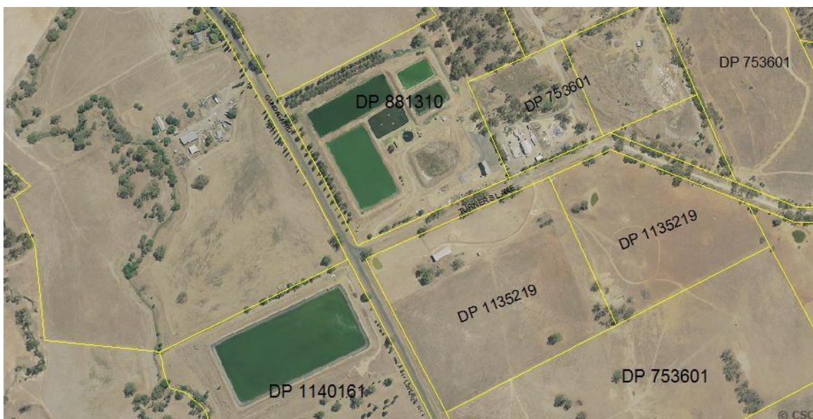
Aerial view of Cootamundra Treatment Plant and surrounding properties.
