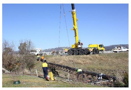
Pictured: Replacing the bridge structure supporting Cootamundra's sewerage and water mains is in progress in Betts Street Cootamundra.
