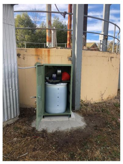
Pictured: The recently installed "Odour Warrior" at the Betts Street sewer pumping station in Cootamundra.
