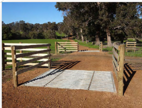
Stock grids along rail trails, such as this one on the newly opened extension of the rail trail south of Margaret River in WA, can allow stock crossings to be open 24/7 thereby enabling stock and machinery to cross the trail unimpeded.
