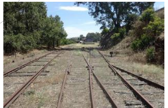
Some of the multiple railway lines will need to be removed to make way for the proposed path.
