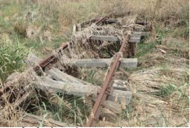
Several short new bridges will be required along the proposed path, replacing the old timber structures.
