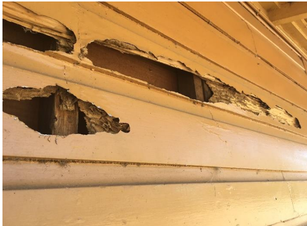
Figure 27: Termite damage
