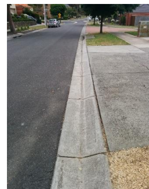
Figure 32: Roll kerbs tend to be longer lasting as they are fully mountable
