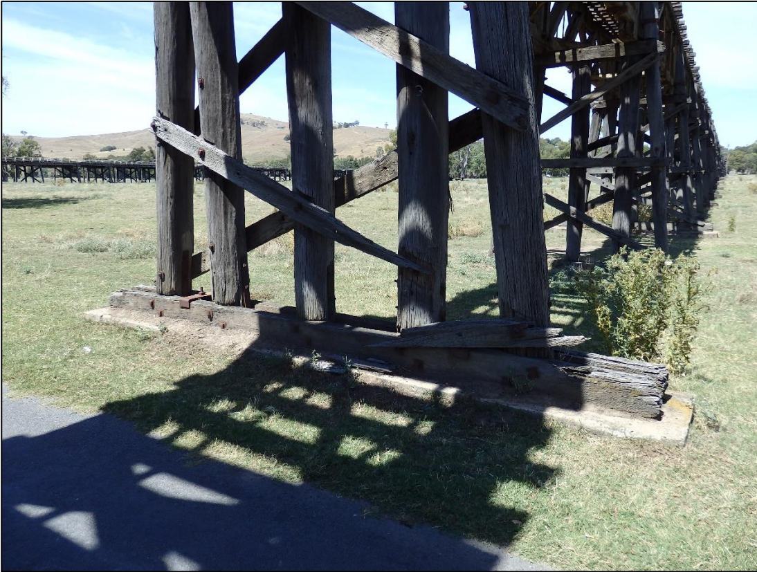
Plate 8 – Broken Lower Cross-Bracing, Trestle 23
