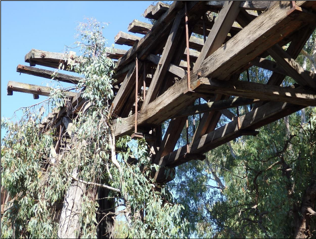
Plate 1 – Fractured Top & Bottom Chords, Span 4, Down Side Truss (near Trestle 4)
