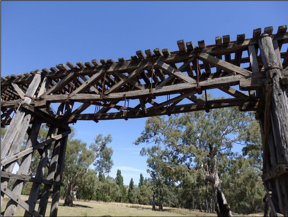
Plate 3 – Fractured Bottom Chord, Span 51, Up Side & Down Side Trusses
