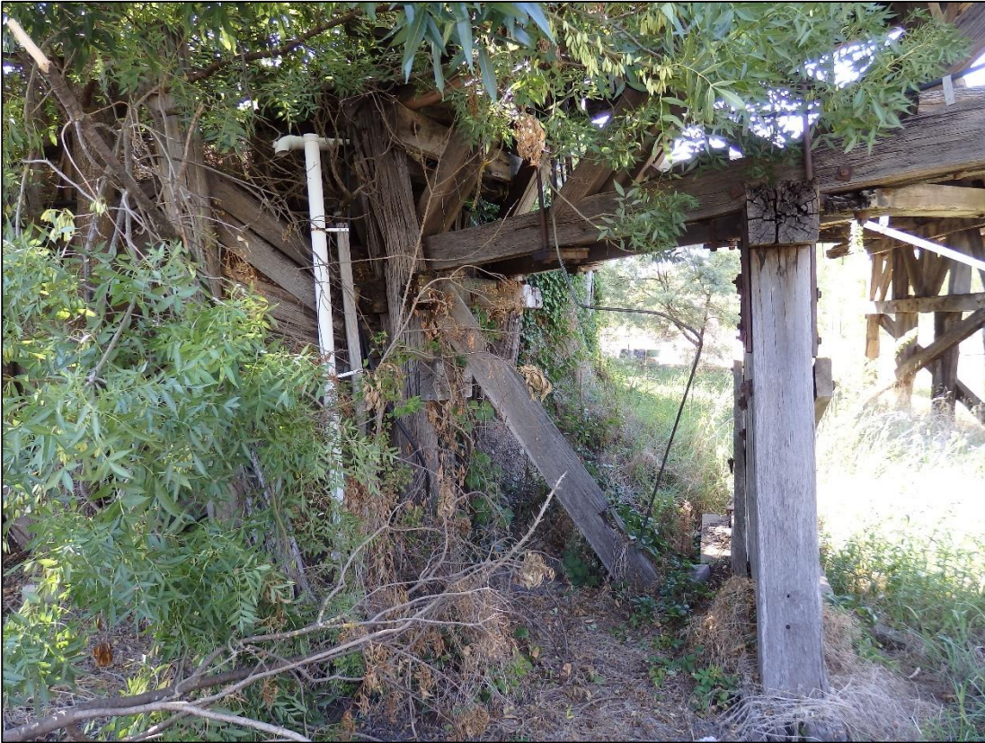
Plate 12 – Dilapidated Abutment 1
