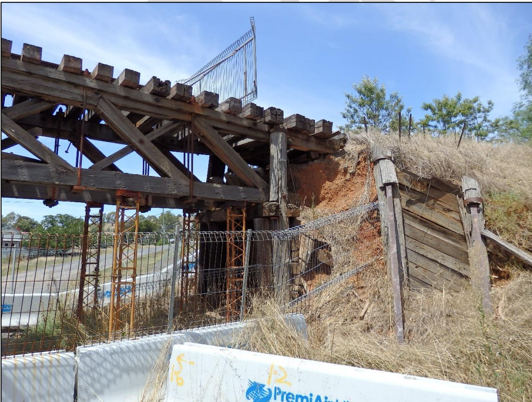
Plate 19 – Dilapidated Abutment 1
