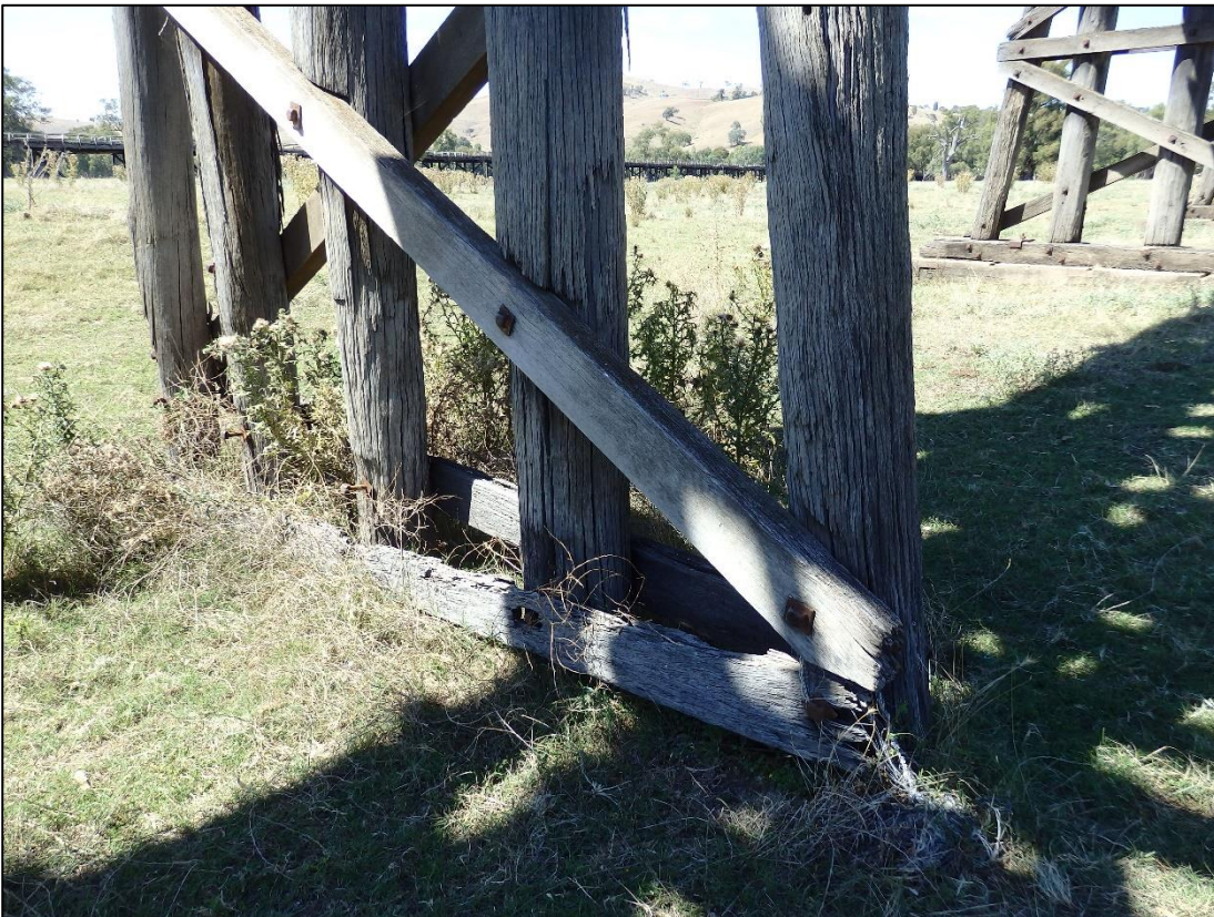
Plate 9 – Severely Deteriorated Bottom Waling, Trestle 26
