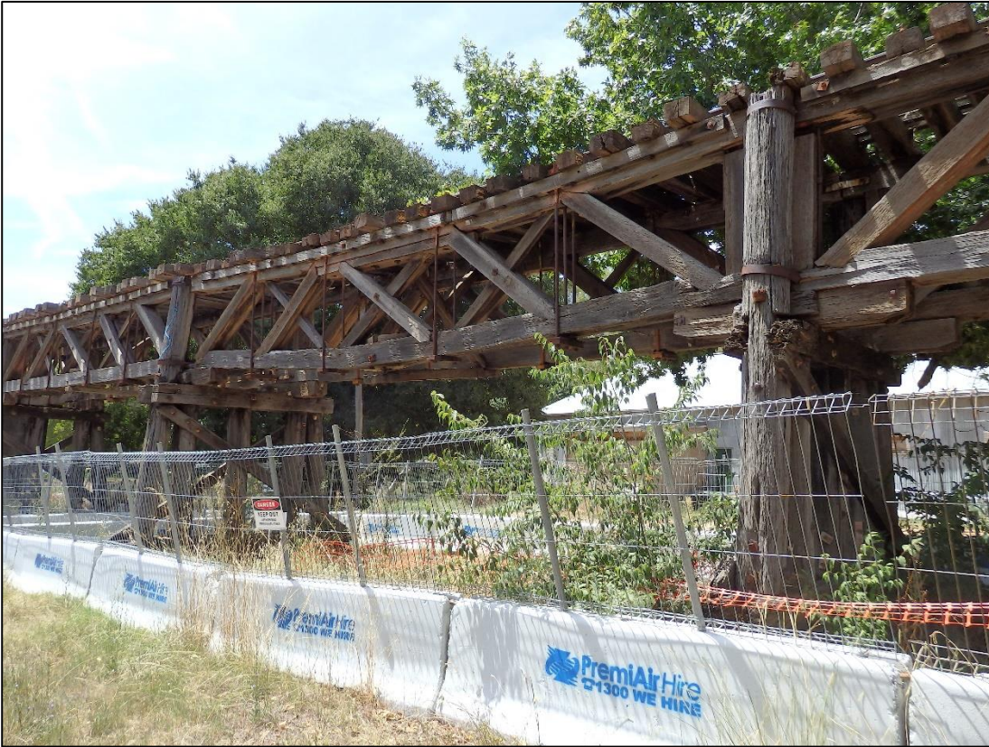
Plate 16 – Sagging Up Side Truss, Span 78
