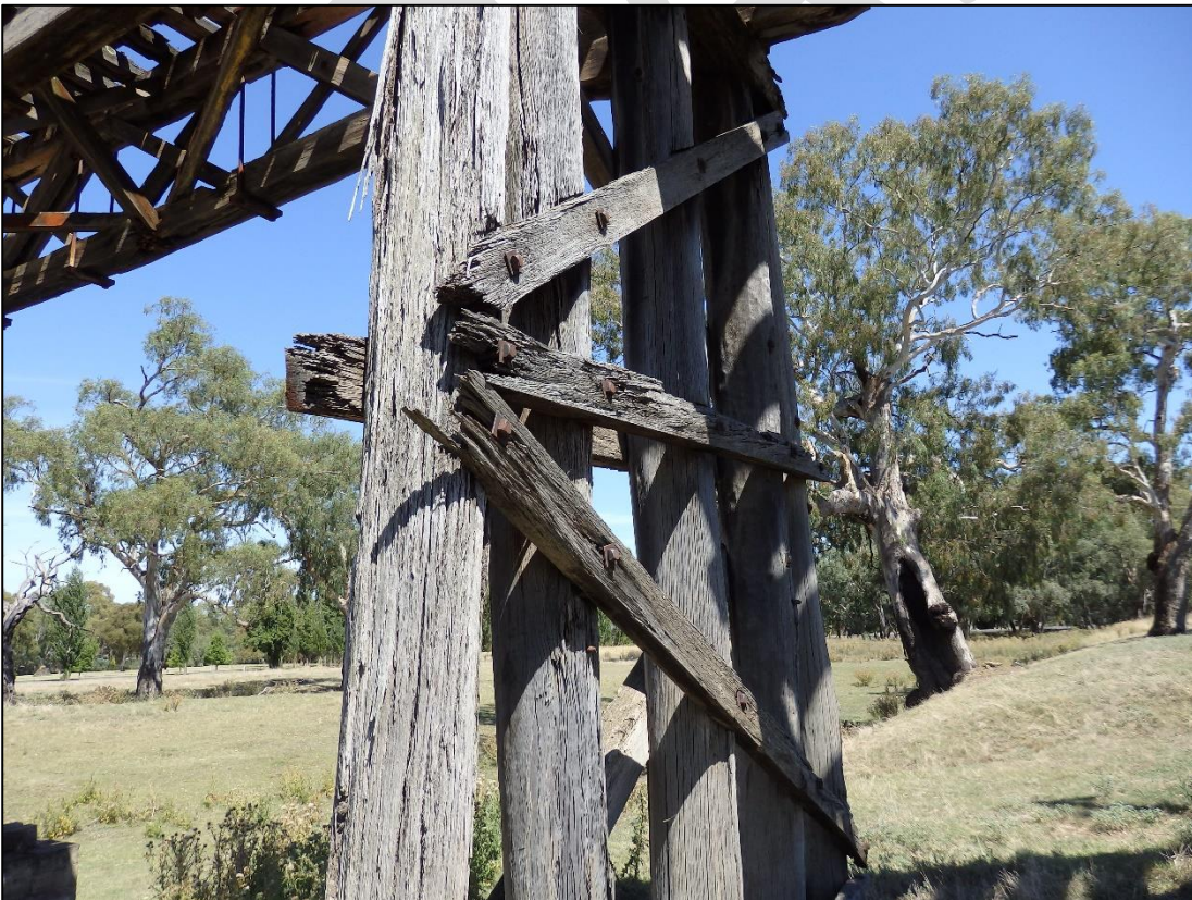
Plate 11 – Deteriorated Mid-Height Walings, Trestle 50
