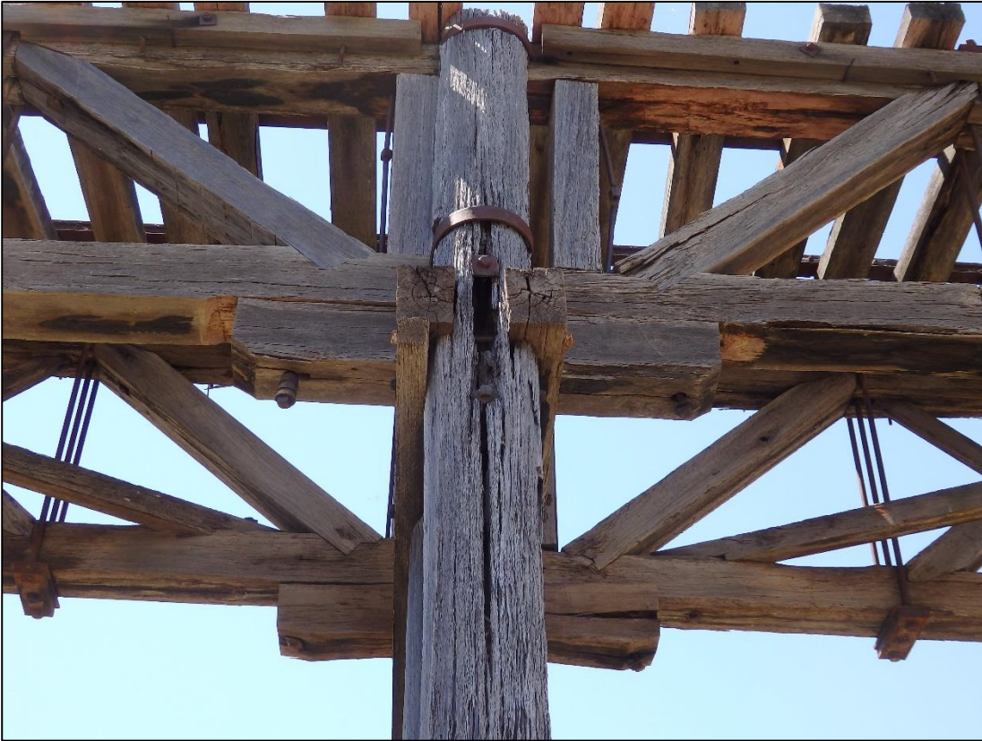
Plate 10 – Split & Decay, Down Side Pile, Trestle 39
