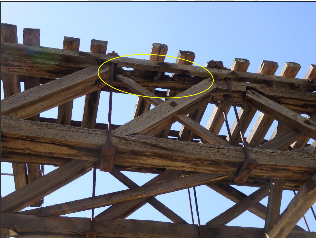
Plate 2 – Severe Decay at Top Chord, Span 25, Up Side Truss
