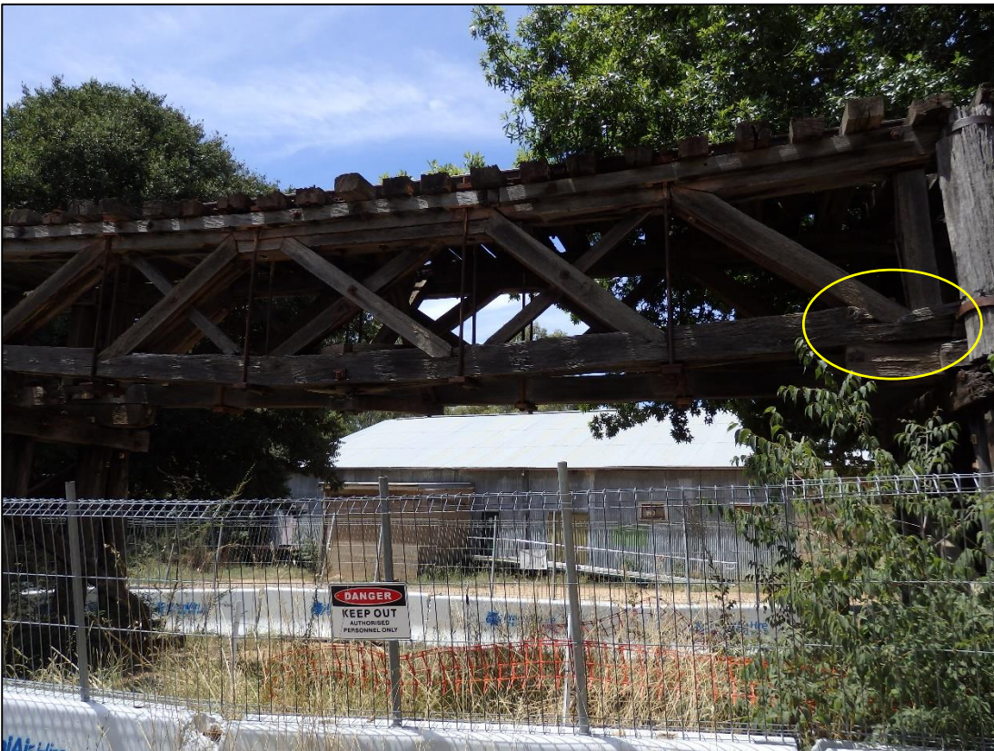
Plate 17 – Bottom Chord Crushed, Up Side Truss (near Trestle 78), Span 78
