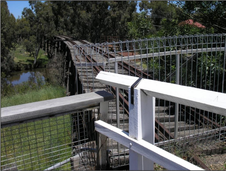
Figure 5 – Top of Typical Timber Viaduct Spans
