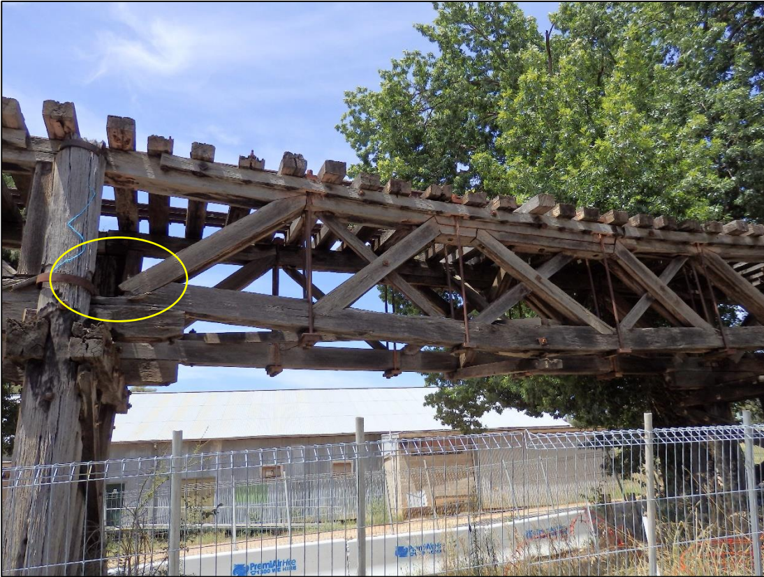
Plate 18 – Bottom Chord Decayed, Up Side Truss (near Trestle 77), Span 78
