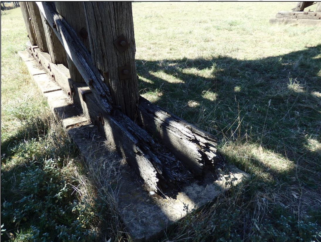
Plate 7 – Decayed Bottom Walings (Typical for Trestles 17 to 22 (inclusive))
