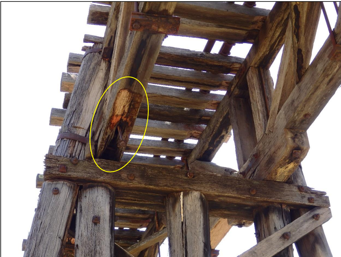
Plate 4 – Missing Corbel & Bottom Chord Decayed, Span 54 (at Trestle 53), Up Side Truss
