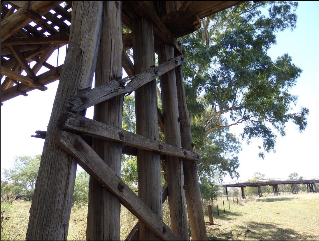
Plate 5 – Decayed Upper Cross-Bracing, Trestle 16
